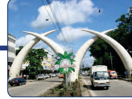
Kenya: Integrated Strategic Urban Development Plans for Cluster 1 Mombasa Town, World Bank funded Scope: Integrated Strategic Urban Development Planning & Capital Investment Planning
