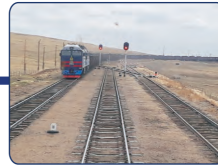
Mongolia: Bogdkhan Railway Bypass Investment Program - 01 (Length: 166.44Km, including 3 Tunnels of Length 15.16Km), ADB funded Scope: Alignment Study
