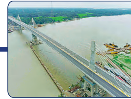
Bangladesh: Paira Bridge (4 Lane, 1.47Km - Extradosed), KFAED funded Scope: Detailed Design, Bid Management & Construction Supervision
