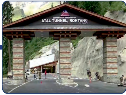
India: Atal (Rohtang) Tunnel, Length - 9.02Km World's longest Single Tube Bi-directional Tunnel at an altitude of 3000m above MSL Scope: Construction Supervision
