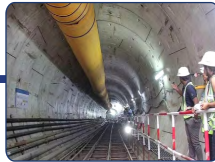
India: Mumbai Metro Line-3, Underground Corridor (UGC-03)(Total Length - 7.57Km TBM Tunnel) Scope: Detailed Design & Design Support during Construction
